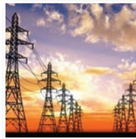
Utilities Power Generation
