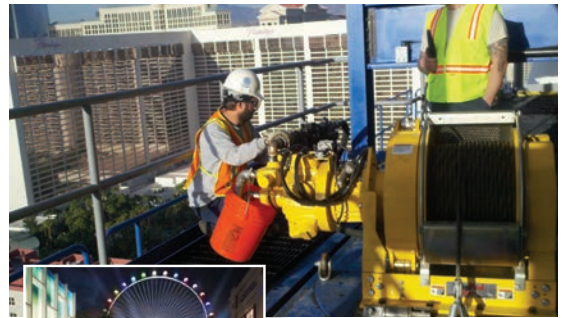
Therm air winch on construction site at Linq project Las Vegas World's largest ferris wheel
